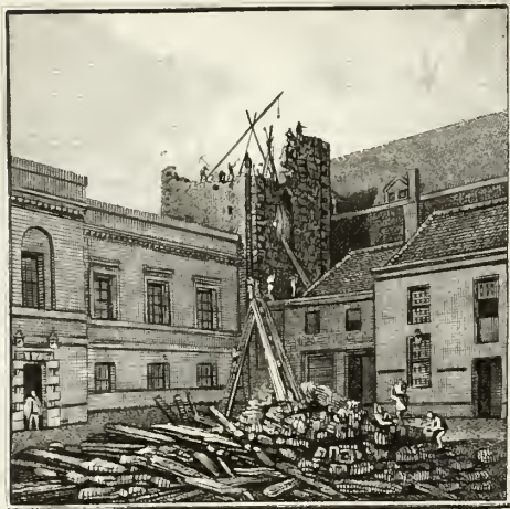
N. E. Side of the Bell Tower of St. Stephen's Chapel
